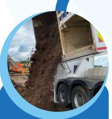
When the skip is full, or once the job has been completed, the excavated material is discharged at the designated location on site.
